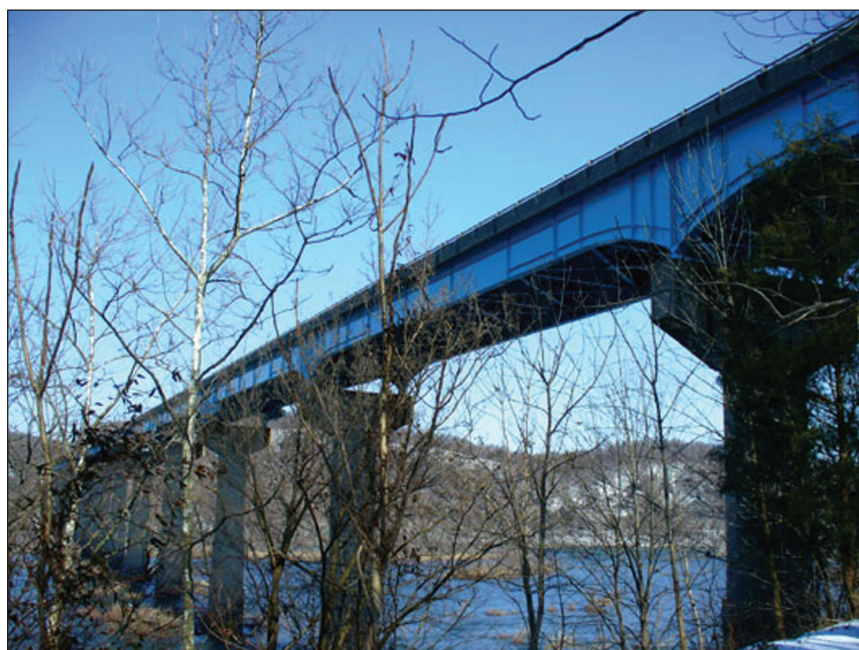
Figure 1. The Norman Wood Bridge (PA-372) over the Susquehanna River.
